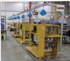
Cable assembly line in Elite's North American facility
